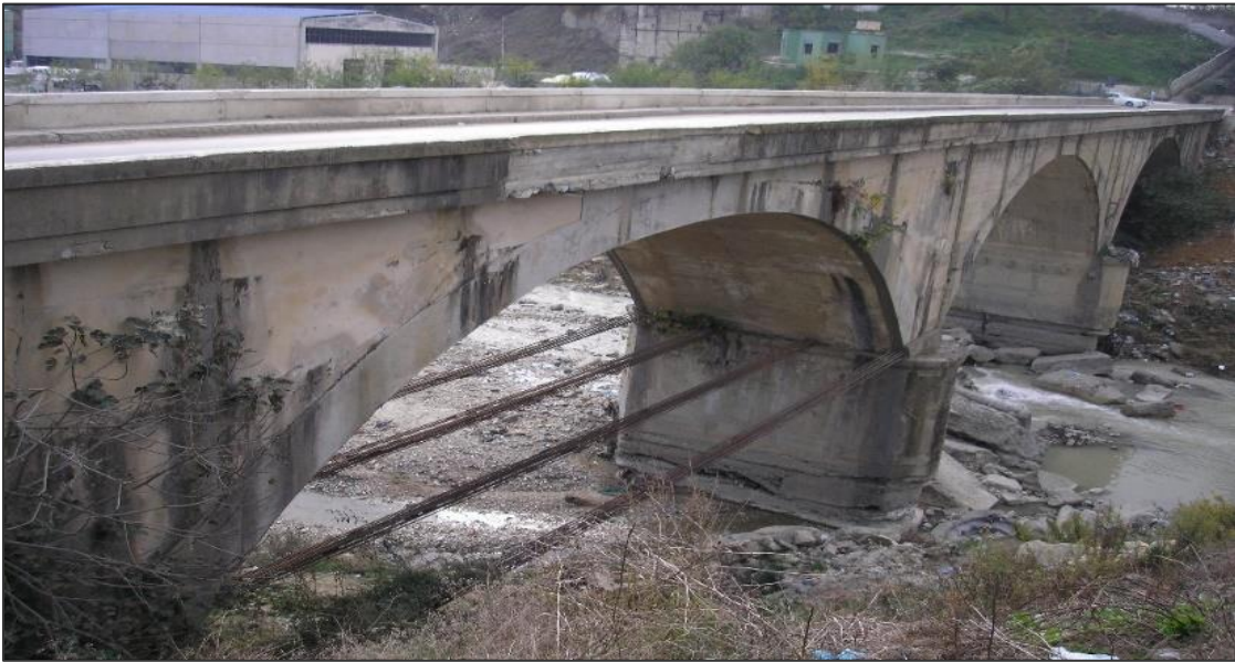
Figure 6: Beshiri Bridge over the Erzeni River – longitudinal view
